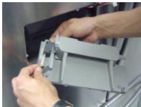
12) Separate the Switch connection harness.
