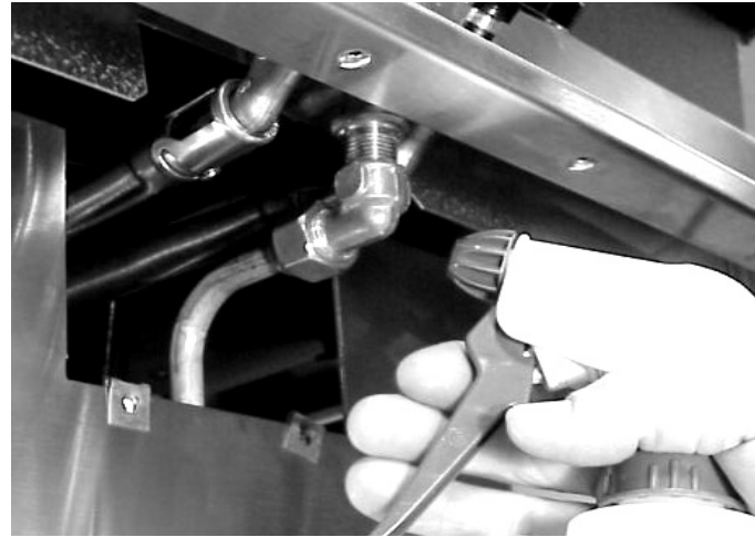
Figure 17 Leak Checking the Valve Connection
