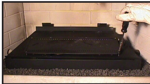
Figure 3 - Burner Assembly
