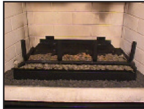
Figure 7 - Rock Wool Placement
