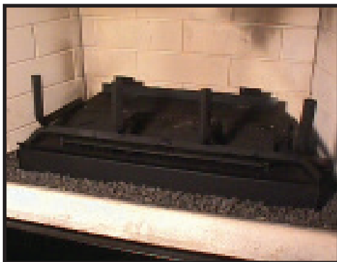
Figure 6 - Placing the Grate Assembly
