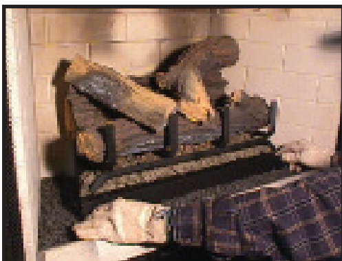
Figure 14 - Access Cover Removal
