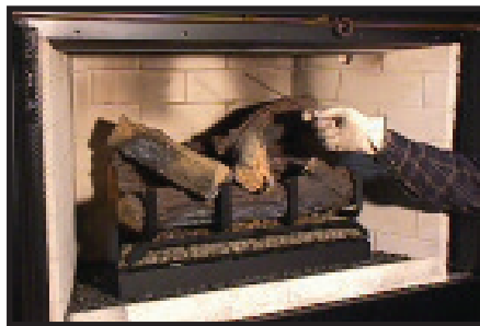
Figure 16 - Checking for Spillage
